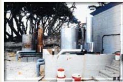
**This sulfurous generator burns elemental S to create  $\text{SO}_3$ , which reacts with water to form sulfurous acid,  $\text{H}_2\text{SO}_3$ .**
